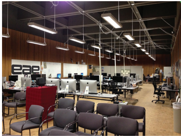
This computer lab at the University of Utah has multiple power and data access points, which not only allows for versatile configurations within the space, but also for easier replacement and upgrading of existing fixtures and technology.
