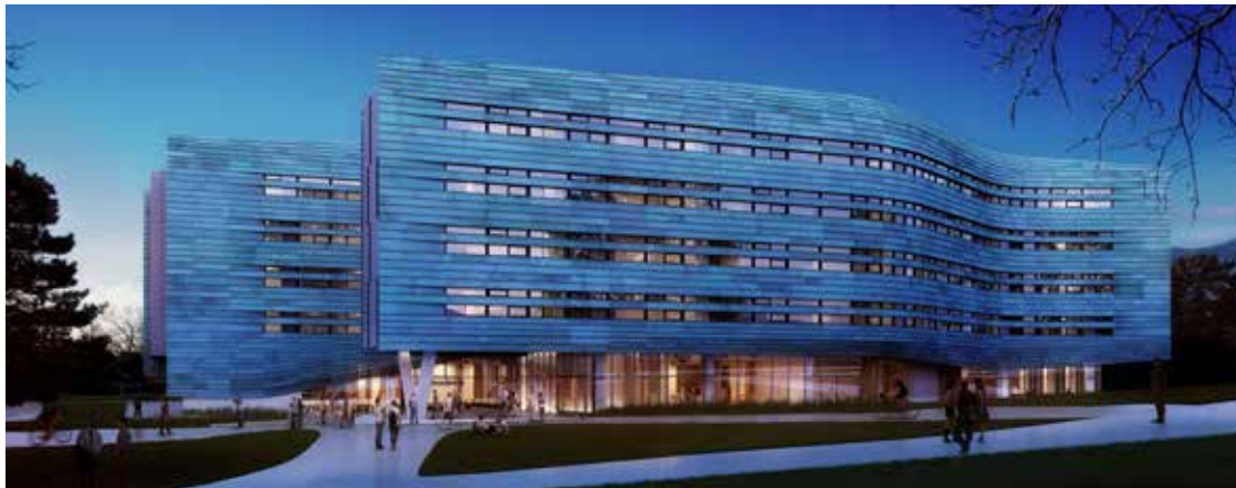
All students will be welcome to "Live. Create. Launch." at Lassonde Studios. (Architectural rendering pictured.)
